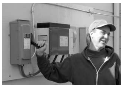
Jon Dixon connects PV system to grid
