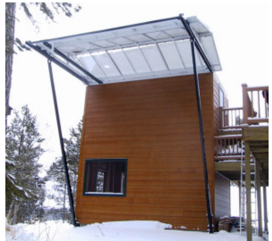
Roof open this spring before the snow finished melting.
