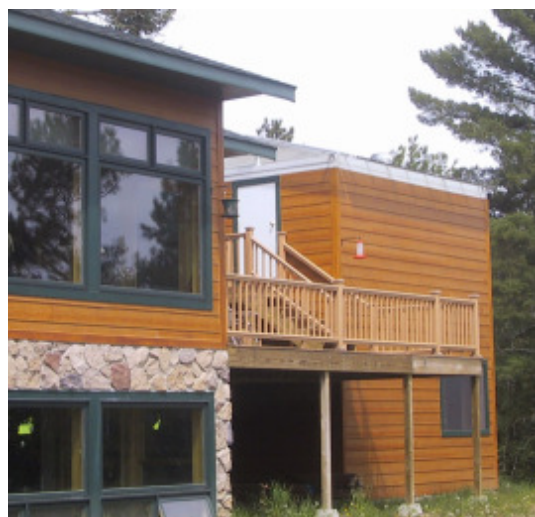
Two views of the observatory, from the east and from the west respectively.
