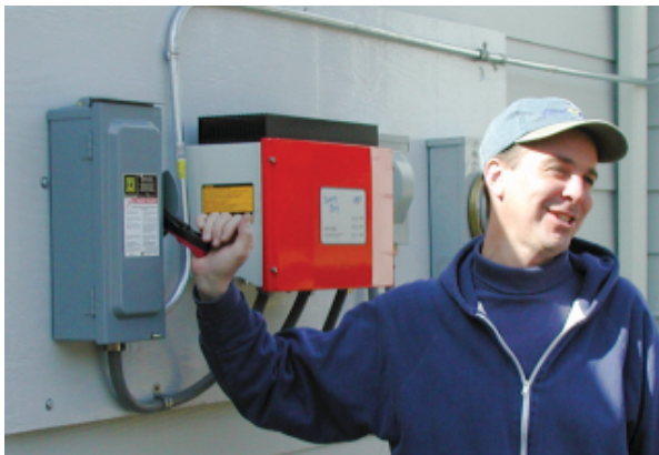
Jon Dixon connects PV system to grid
