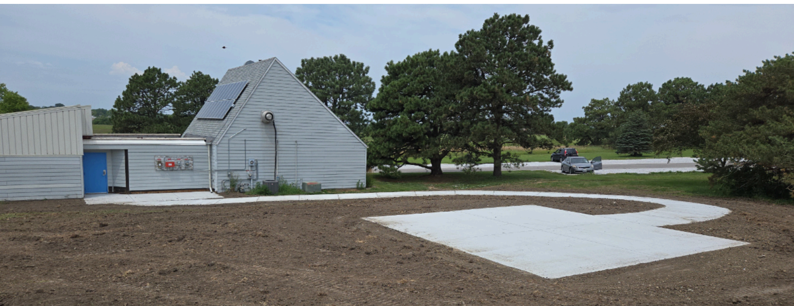
A 16' x 16' pad has been installed on the east side of the observatory
